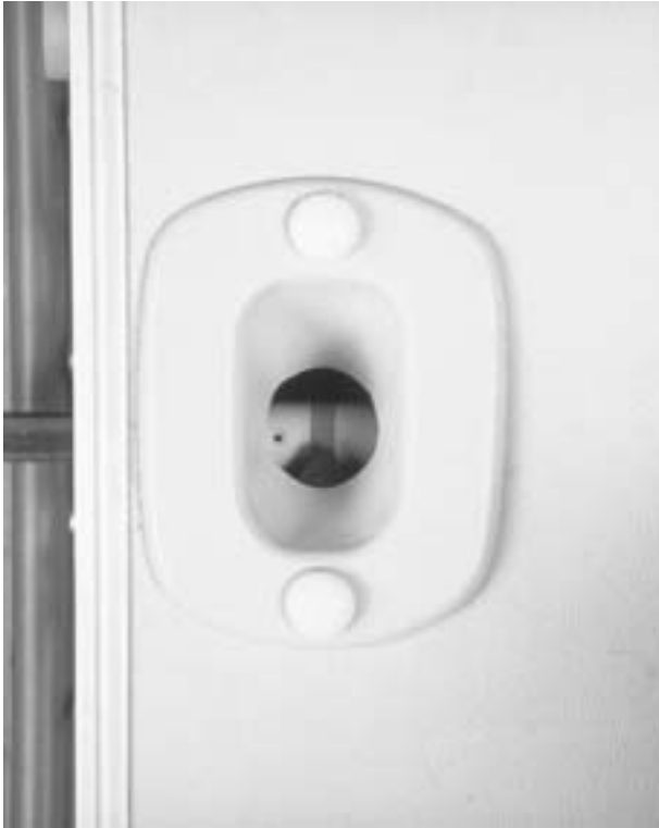
Figure 1-30. Latch Bolt
