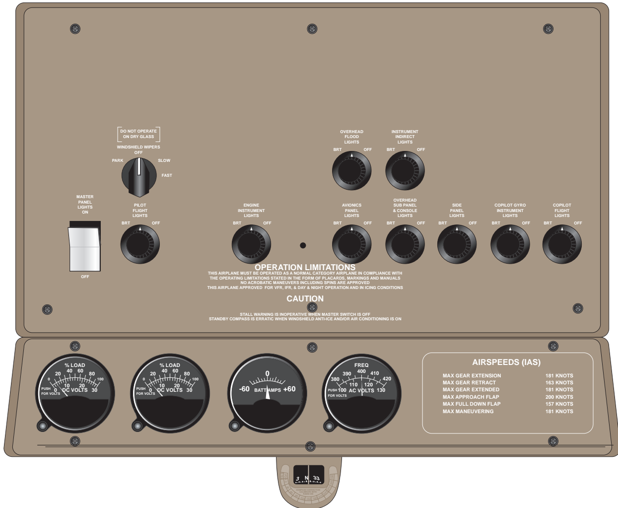
Figure 3-1. Overhead Lighting Controls
