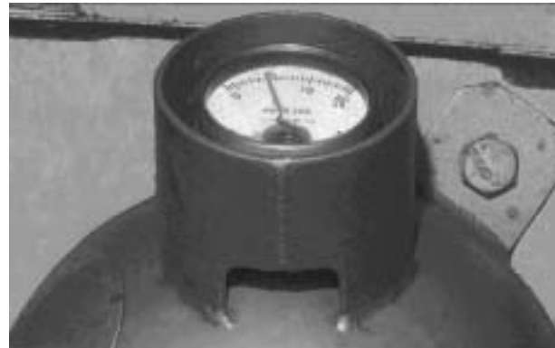
7. FIRE EXTINGUISHER PRESSURE (IF INSTALLED)—CHECK
