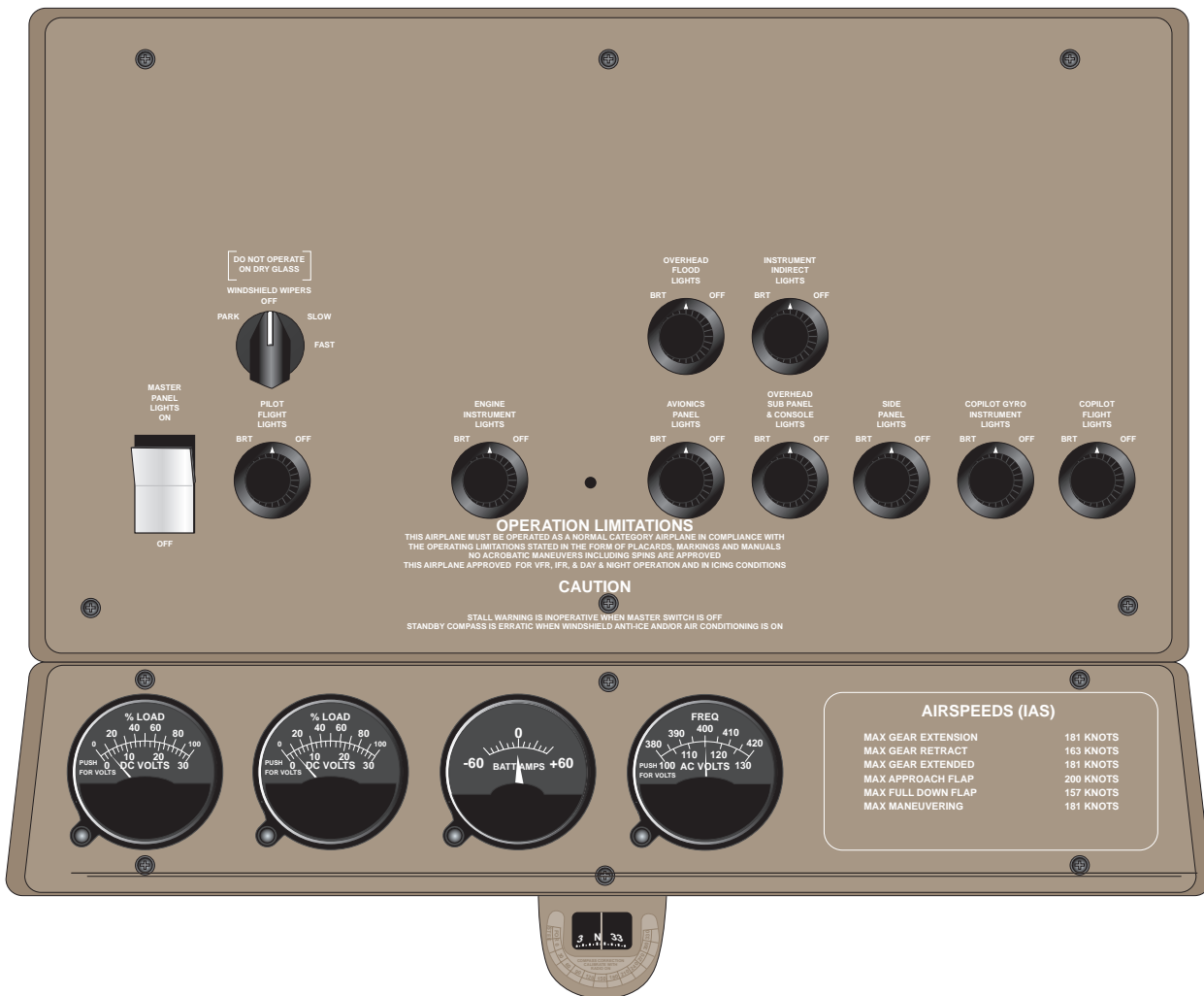
Figure 1-4. Overhead Light Control Panel (BB-1632 and After)
